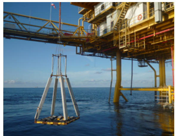
VERY COST-EFFECTIVE RetroPod installation time is only one-fourth that of traditional anode retrofits.
